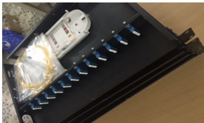
Fig. 1 Splice and termination box
